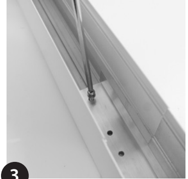
3 Tighten 4x screws.
